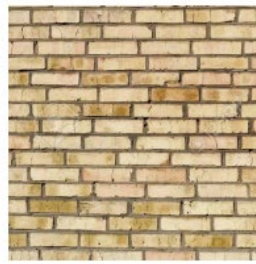
MW-01 Existing brick to be stripped
